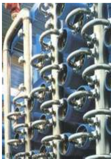
END PORT installation
