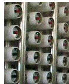
SIDE PORT installation
